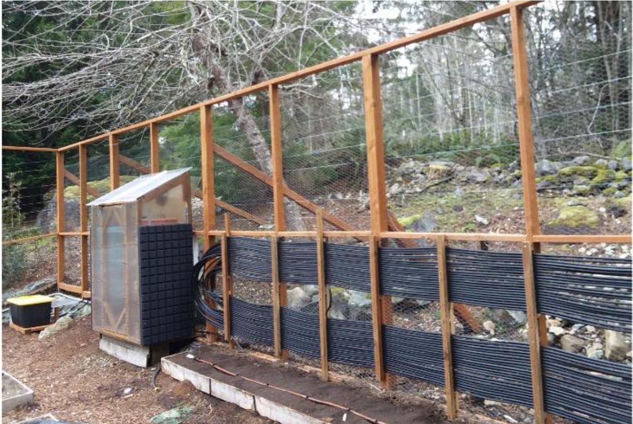
Figure 373 Solar Collection Water Tubing
